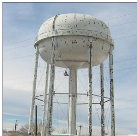
BEFORE – The Zuni Water Tank before repairs and rehabilitation.
